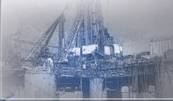
Oil & Gas / Petrochemical Öl- & Gasindustrie / Petrochemie
